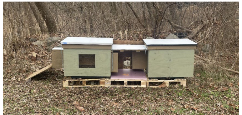
Figure 2. New cabins and feed station installed at business.
